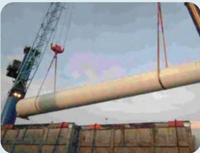
Towers being loaded in Bremerhaven Port, Germany
